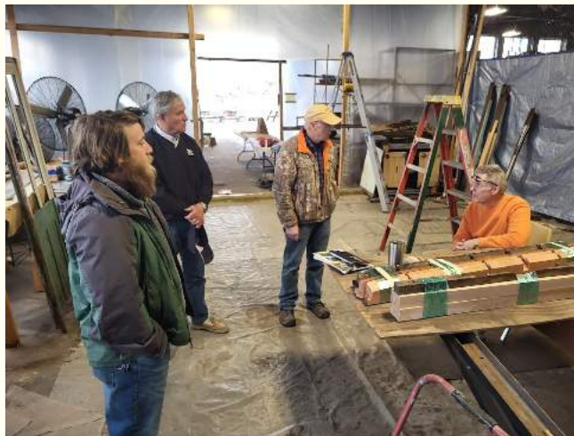
Photo of TWWWG members delivering parts needed to reconstruct portions of a curved wall on the Hampton streetcar.
